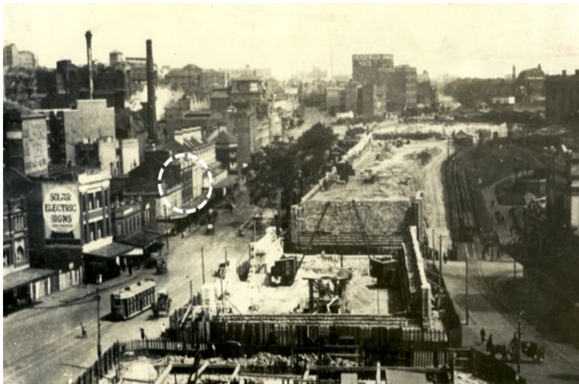
Figure 3-26: 1925 During the construction of Central Station (Source: City of Sydney Archives A-00006195< https://archives.cityofsydney.nsw.gov.au/nodes/view/566840 > )
