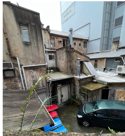
Figure 4-6: Rear of Buildings part 238-40, 232-236 Elizabeth and rear yard from first floor (Source: Curio 2022)
