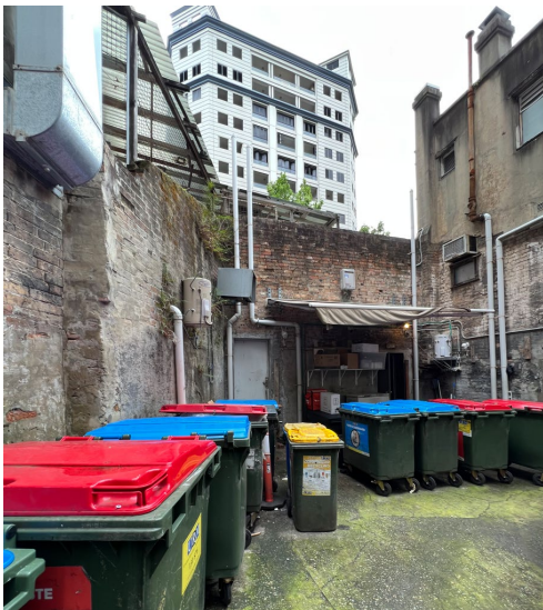
Figure 4-5: Rear of buildings 238-40 , infill and rear yard from ground level (Source: Curio 2022)
